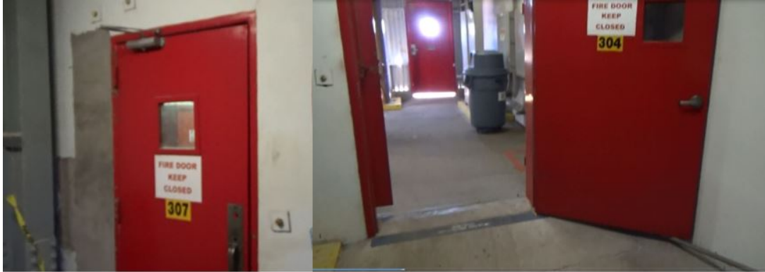
Figure 3. Doors within the manufacturing building on the 3 rd floor that separate the east (wet end) and west (dry end) sides. Although intended by design to remain closed, these doors were propped open at times, as shown in the photograph of door 304 on the right.
