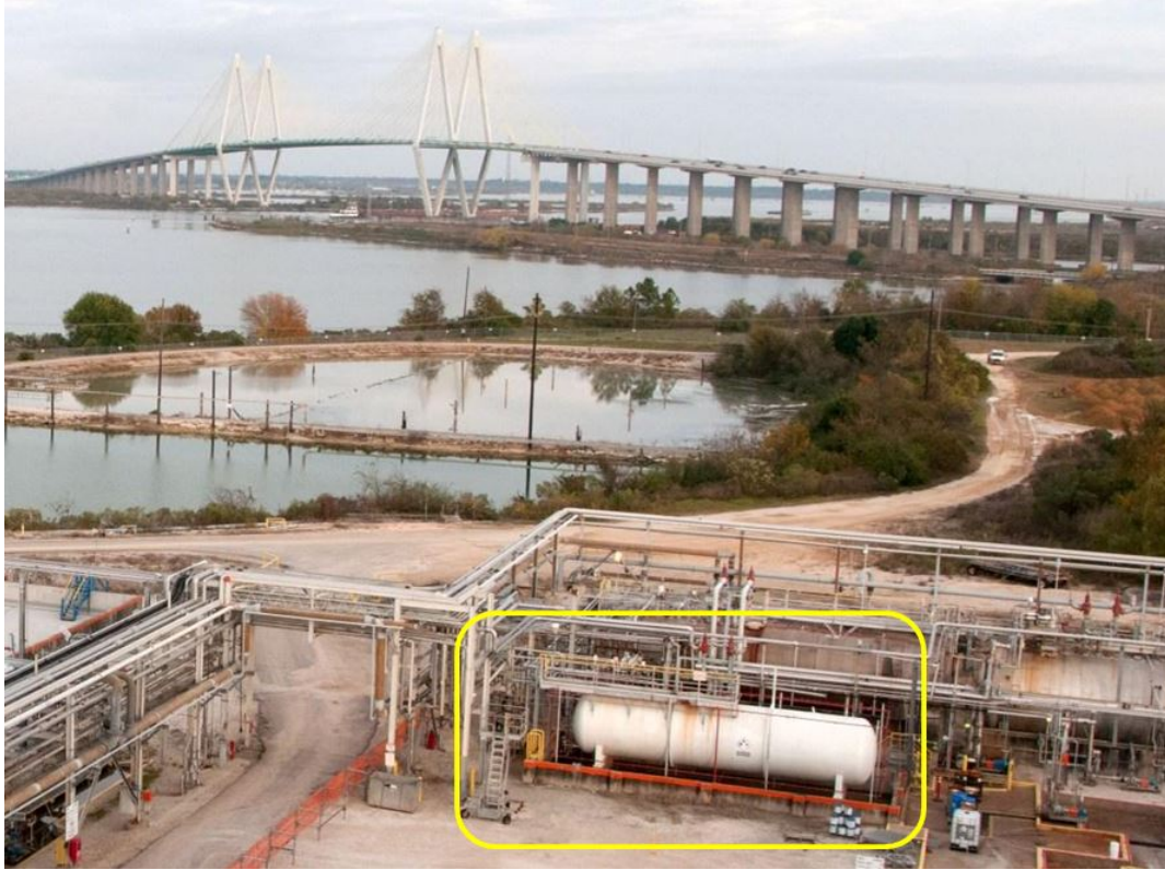
Figure 13. The yellow box outlines the 18,000 gallon methyl mercaptan storage tank at the DuPont facility in La Porte, Texas. Both the Lannate ® and Vydate ® insecticide processes use methyl mercaptan as a key raw material.
