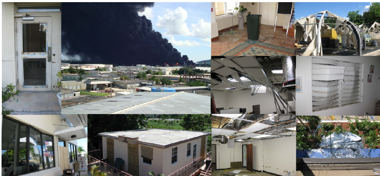
Figure 10: Community damage surrounding the CAPECO facility
