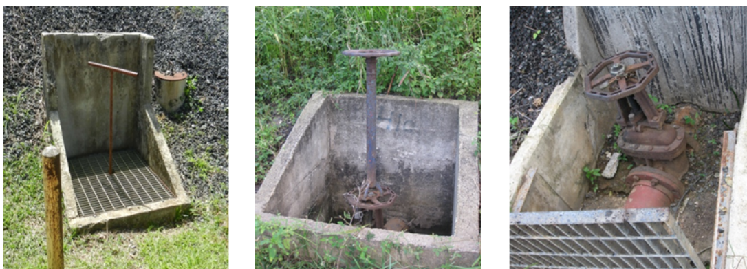
Figure 15: Various dike drain valves at CAPECO. Tank 409 dike drain valve (left): position of the valve is undeterminable without physically turning the valve. Rising stem valves (center, right). In some cases, the valve position is hidden in the sump (center).
