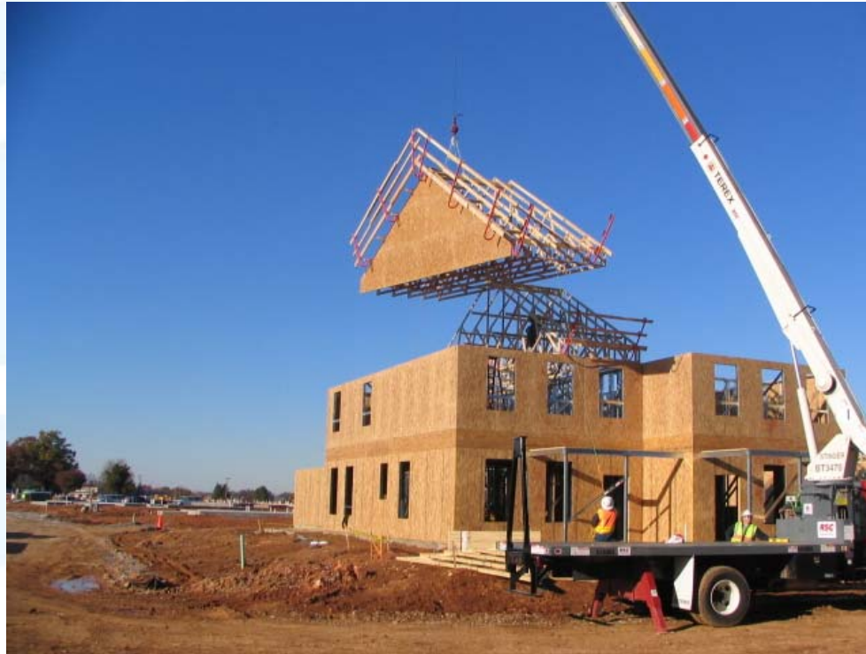
Pre-installed fall protection
