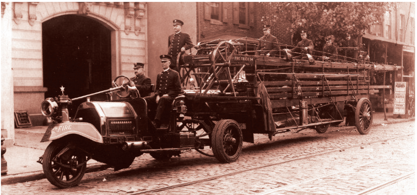
Photo Courtesy of the Philadelphia Fire Department
