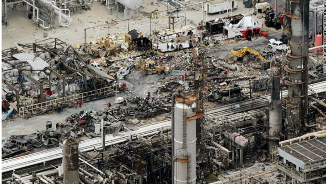
Figure i. The aftermath of the 2005 BP refinery explosion in Texas City (Photo: CNN)
