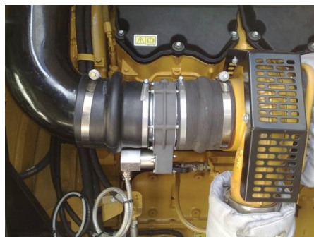
SVX Failsafe Install
