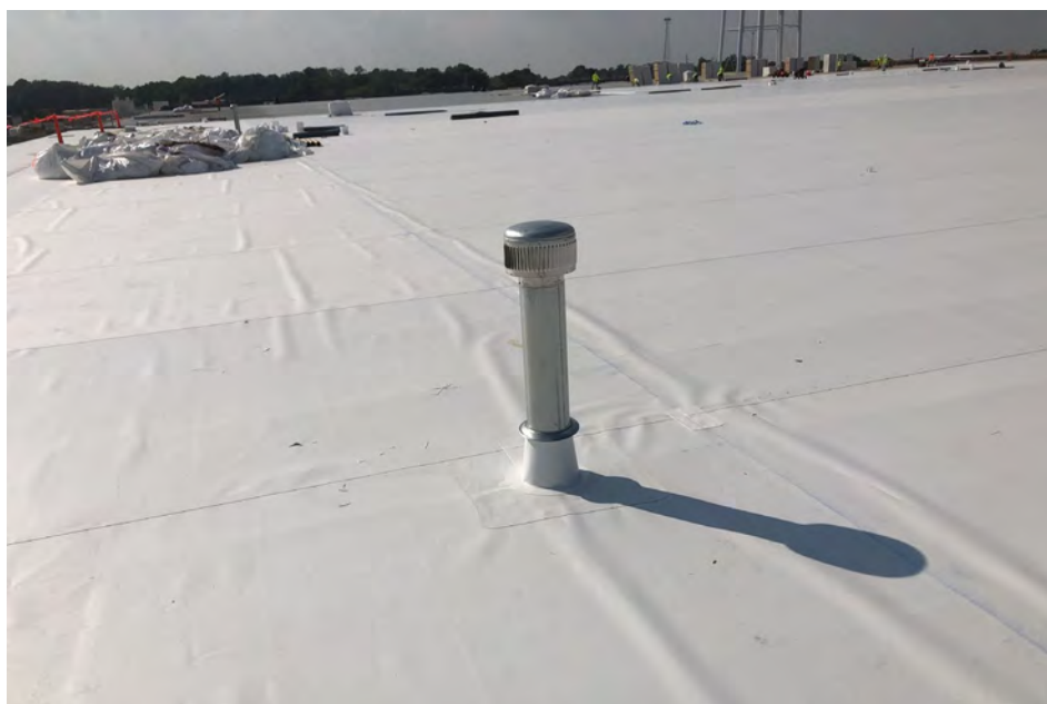
Figure 30. Roof penetration at the Plant 12 Storage Warehouse. (Credit: ARCO)
