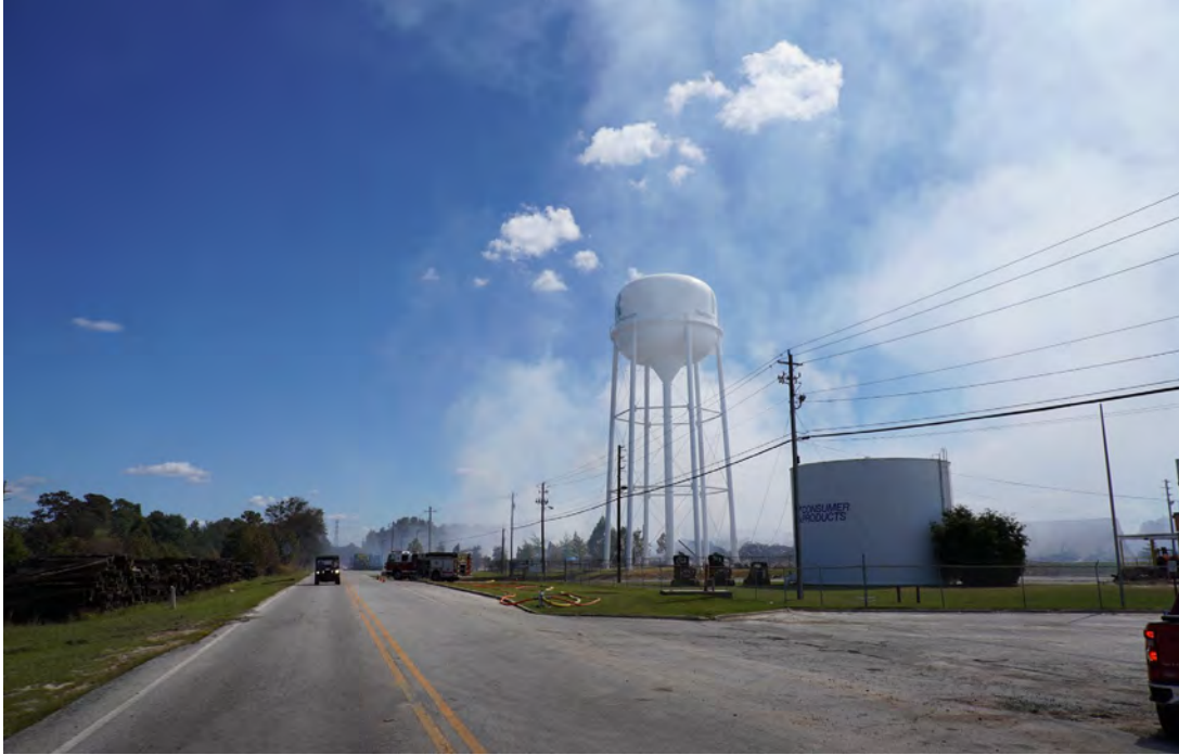
Figure 26. Ongoing off-gassing observed from the site during cleanup operations on October 2, 2024, several days after the incident. (Credit: CSB)
