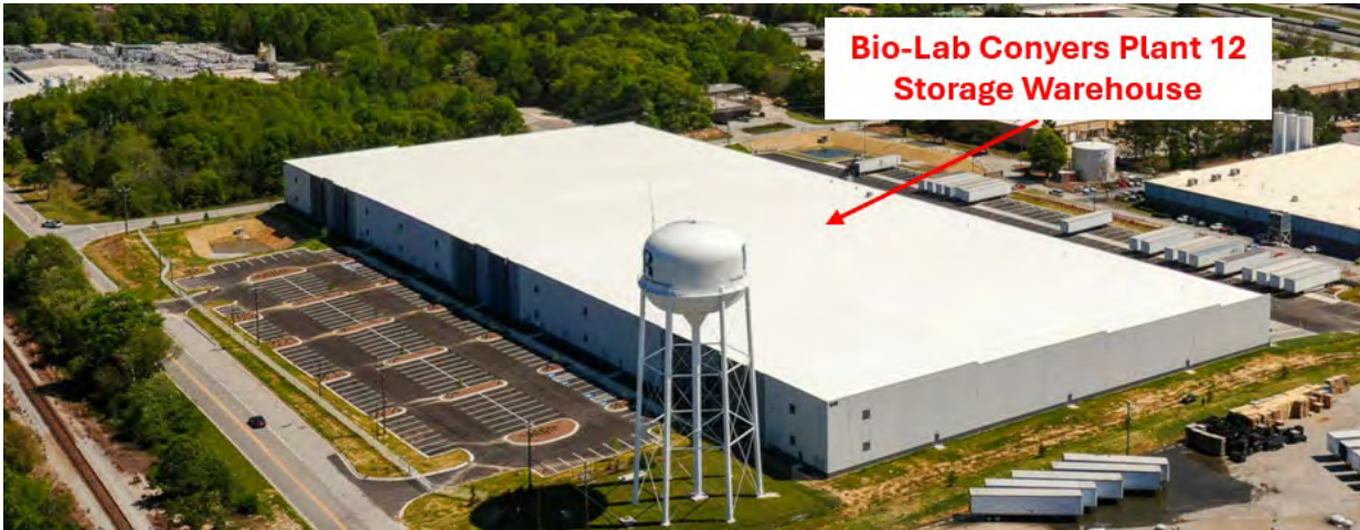
Figure 3. The Bio-Lab Conyers Plant 12 Storage Warehouse. (Credit: ARCO, annotated by CSB)
