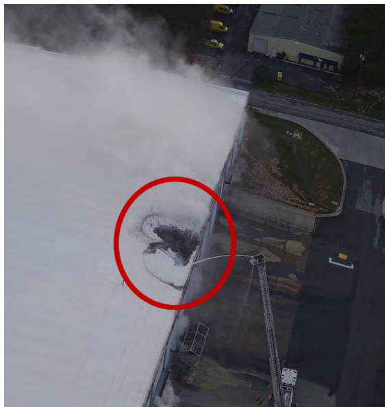
Figure 41. Location of the roof fire (red circle) resulting from the single-point heat source developed outside the bunker, in front of the fire barrier wall at Plant 12 Storage Warehouse. (Credit: CSB)
