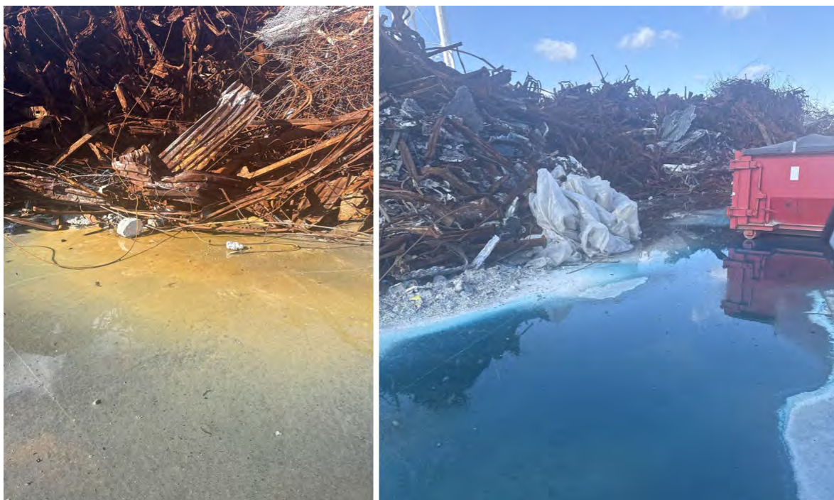
Figure 28. Surface water runoff of metals from rusting structural debris (left) and residual chemicals (right) on the former warehouse’s concrete slab. (Credit: KIK) b
