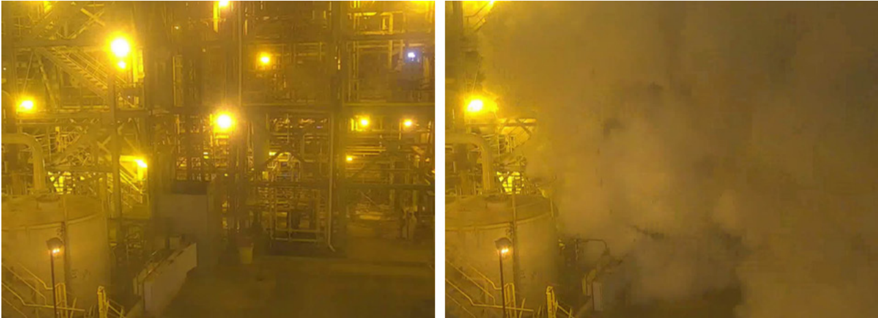
Figure 17. Surveillance images immediately before (left) and four seconds after (right) the reboiler rupture. (Credit: Honeywell)
