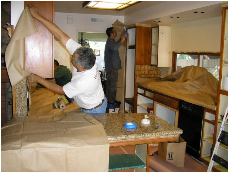
Figure 3-14. Workers Preparing Kitchen for Stripping
