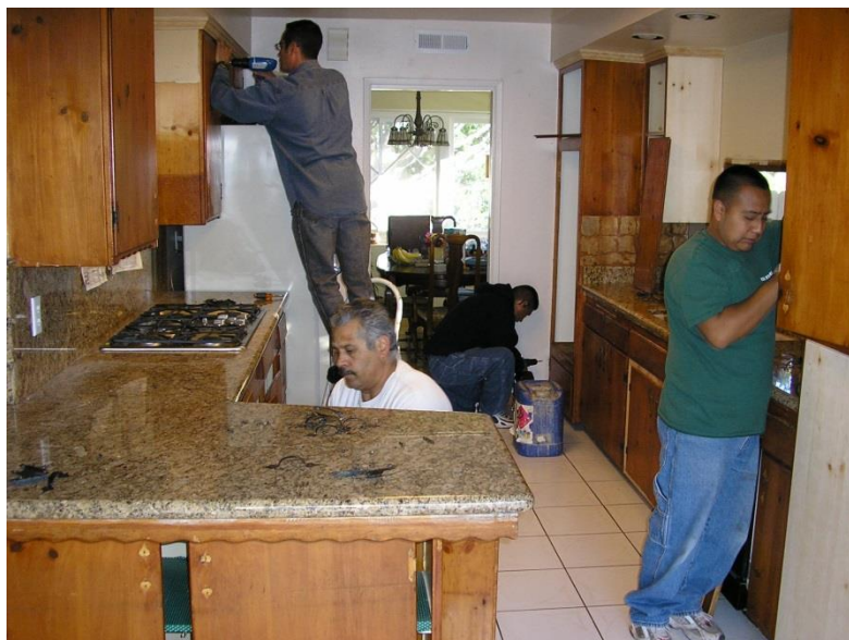
Figure 2-3. Preparing Kitchen for Stripping
