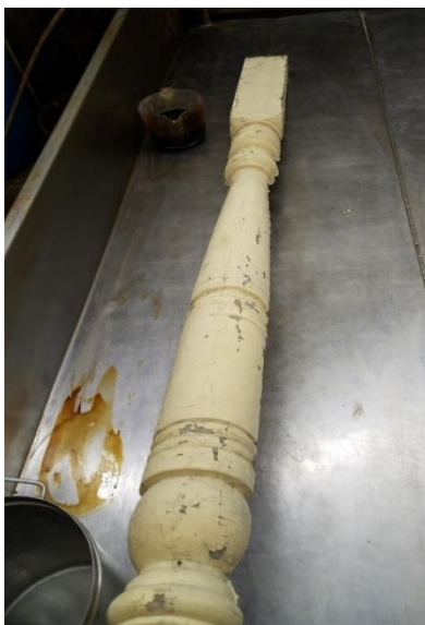
Figure 2: Decorative column with lead-based paint
